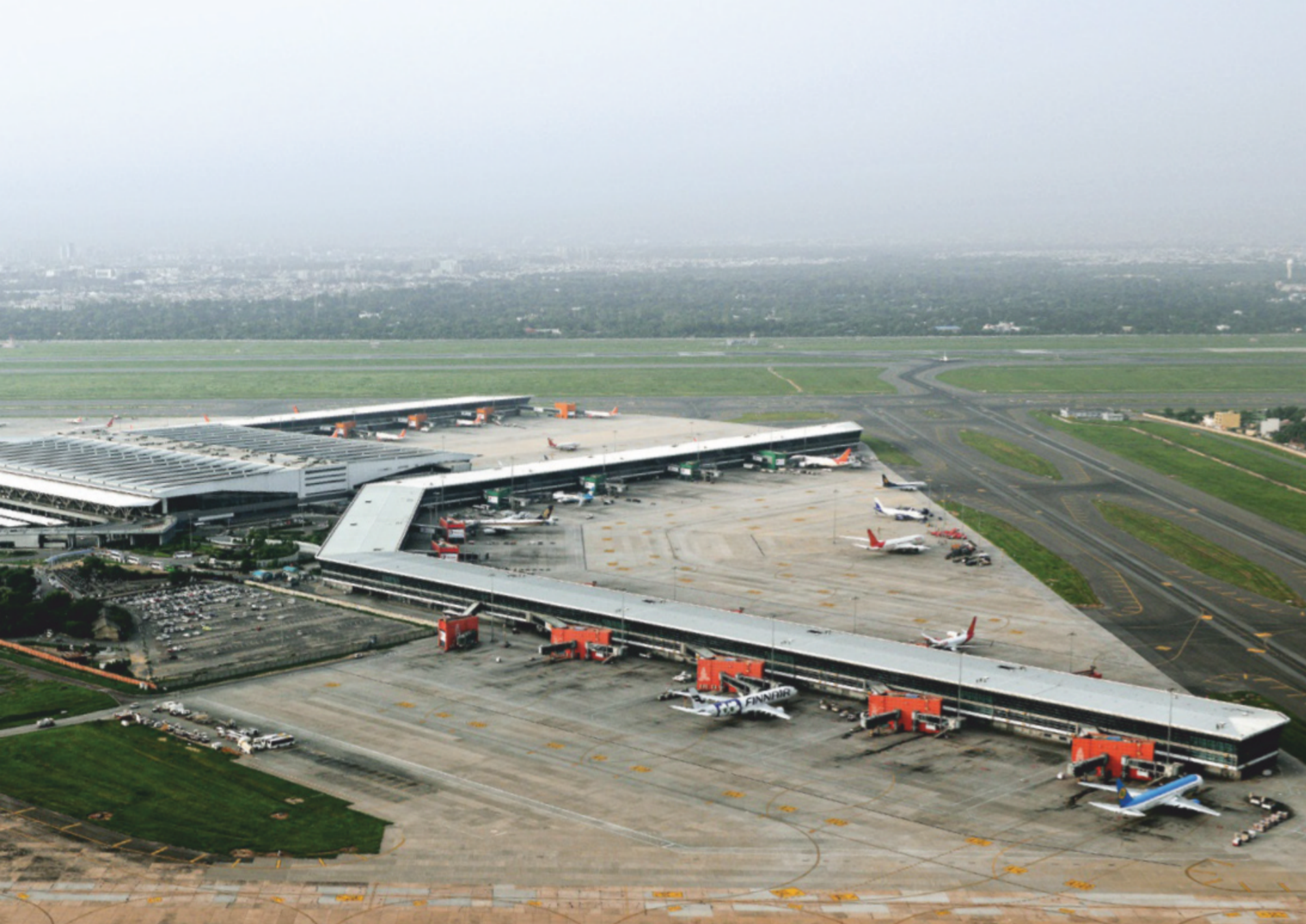
Timely decision on a master plan for Delhi airport (in picture) would have meant India becoming a regional powerhouse in aviation
